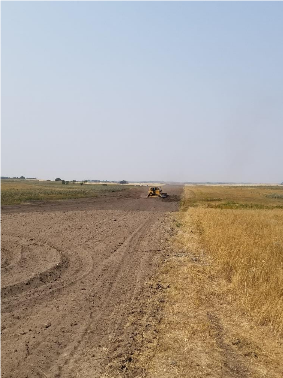
Last dozer in High Pound hill moving a rare plant pile and levelling.
