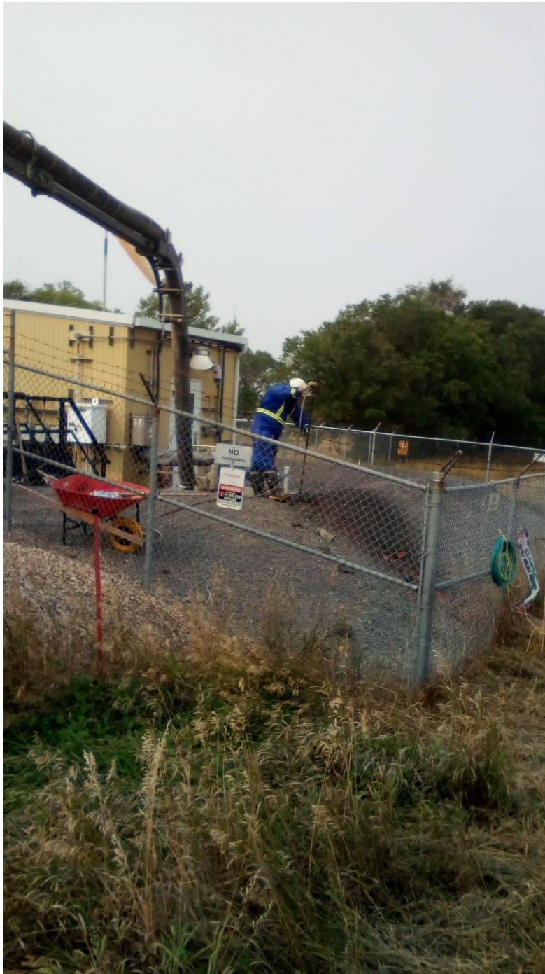
Installation of Cathodic protection at Stoney Beach compound.
