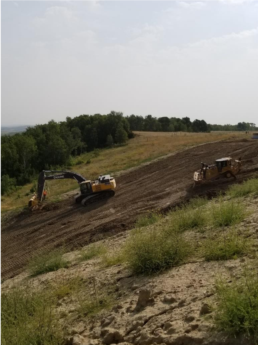
Removal of water diversion berms at Qu'appelle valley.
